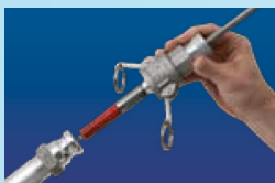
Drill Access Hole in Elbow or Pipe
