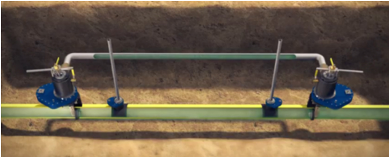
Fig. 5 Still Image of PE Line Stopping System
